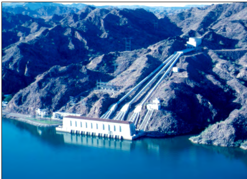
Figure 3. Metropolitan's Whitsett Intake Plant. The plant pumps water from Lake Havasu to the Colorado River Aqueduct, 49 for distribution to 23 of Metropolitan's 26 member agencies. 50 Source: The Metropolitan Water District of Southern California
